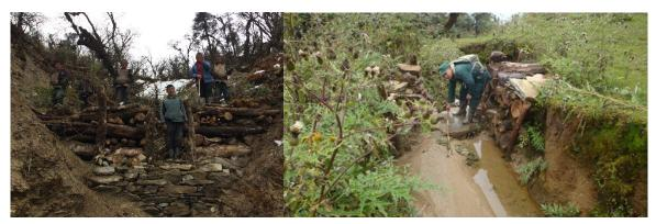
Figure 1 Checkdam construction and sediment control at Drana Gully
